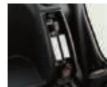
Central fuse box located behind seat
